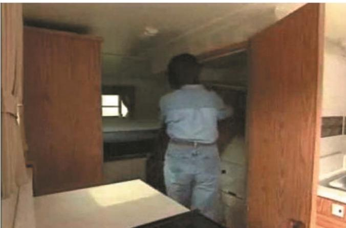
**Step 15:** Grasp the rear and side bathroom walls in the middle of the top edges and lift together toward rear of trailer.
