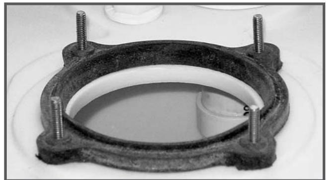
16. Place toilet on studs and secure with four washers and four nuts.
