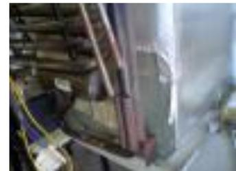
inside the large tube. The two electrical heating elements merely sit in a round tube of there own. All of these vertical heat tubes are welded to the main tube that contains the ammonia gas. The idea here is simple: whatever form of energy is used, it's only function is to apply heat to this area of the tube with the ammonia gas. The insulation is only used to concentrate the heat in one area and to keep ambient air from cooling off this area.
