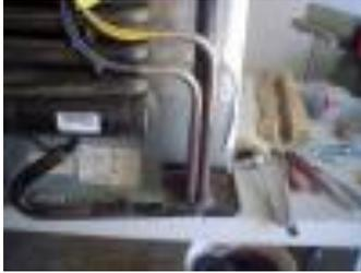
You can begin by carefully cutting the aluminized foil wrap around the insulation. Look at the next photo and you will see that this insulation is really two half round pieces that are held together by nothing more than the aluminized foil. You can see or feel exactly where the pieces join together. Use a razor blade or sharp knife to cut right along this joint. Remove the two halves of insulation to
