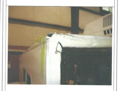
10. Retrieve a second triangle seal (reference step 6). Place the triangle seal at the top ODS corner of the rear seal (closed side of the seal faced down) and staple in place with a N10BAB staple gun.
