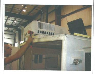
13. Use a rubber mallet to bend the metal sheeting overhang down onto the seal at the rear of the ODS wall frame.
