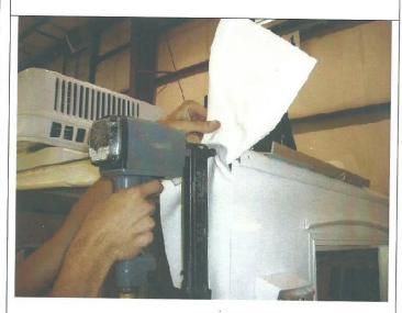
4. Pull the door side (DS) end of the seal on the roof frame out past the side wall and staple it to the end of the frame on the roof and side wall with a N10BAB staple gun. Repeat for the off door side (ODS) end of the seal.
