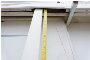
Measure from the bottom of the lift arm inside the pocket stop
