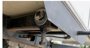
Washer in place
