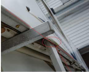
Partial collapse of pocket. Note bulge.
