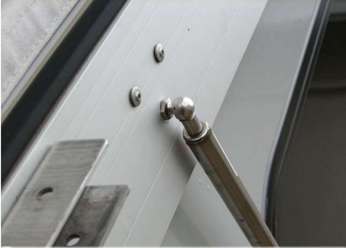
New 10 mm Stainless Steel Ball Stud Placement
