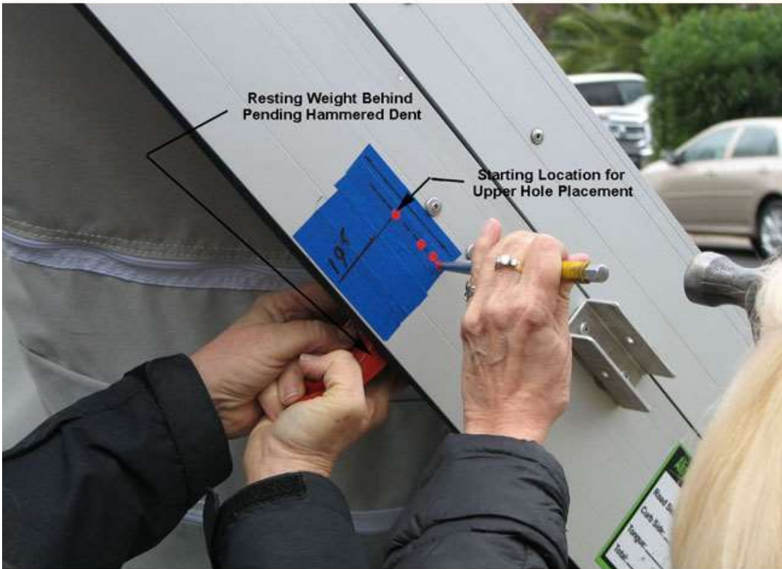
Indenting the Location for the Upper 5/16" Diameter Holes
